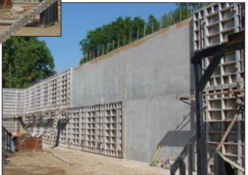
Big Panels stacked to achieve a 16' wall on a commercial project.
