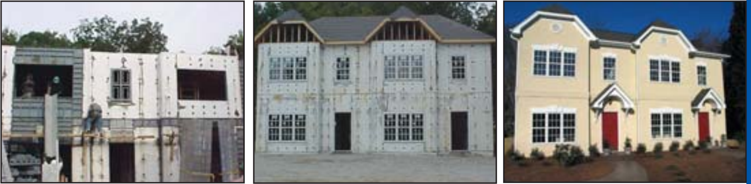
From Stripping of Concrete Forms to Finished Home
