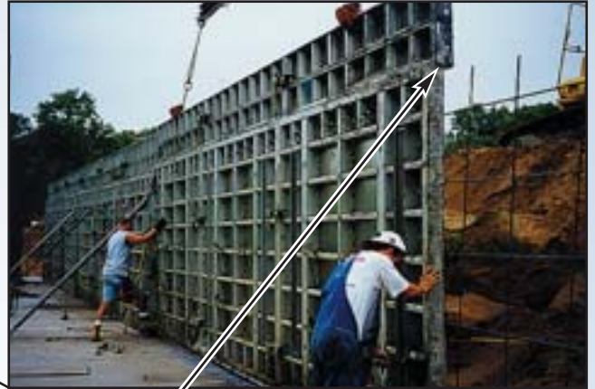
Agricultural project with 2" offset in wall.
